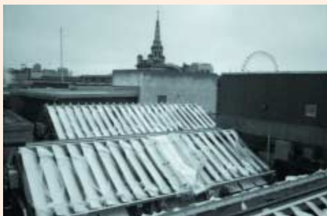
New roof – lights and louvres being installed
